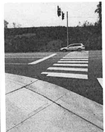
Steele Road at Hardin Valley - Intersection and Roadway Rehabilitation - Knox County
