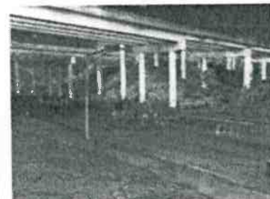
I-24 Bridge over Chestnut Street - Hamilton County
