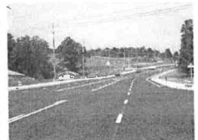
Lovell Road - 2.4 mile widening - Knox County
